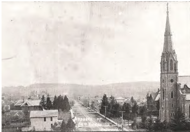
Looking over New Vienna Main Street New Vienna in 1910, looking south.
