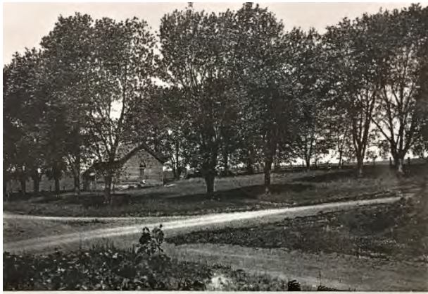
Bloomington School District #2 Thornton School
